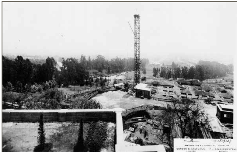
Construction Photo No. 2 Taken 5-9-27
