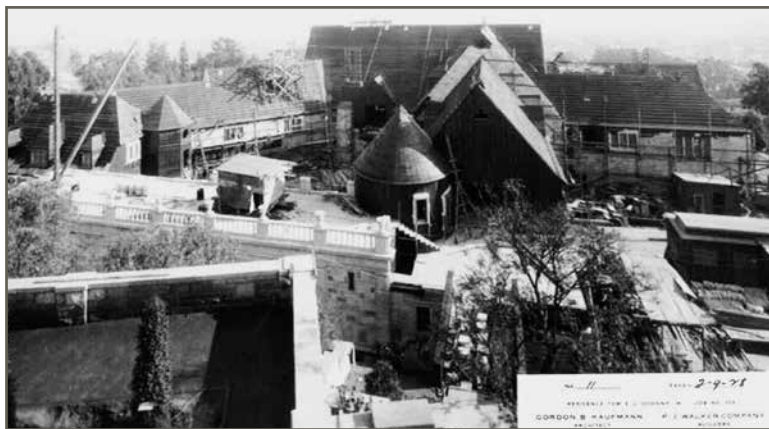
Construction Photo No. 11 Taken 2-9-28
