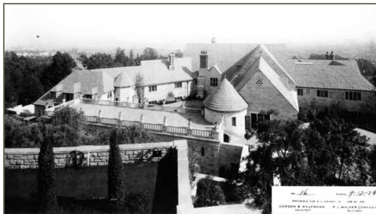
Construction Photo No. 16 Taken 9-12-28
