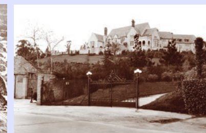
Greystone Mansion and Doheny Ranch Gate entrances side-by-side on Doheny Road/Loma Vista Courtesy of Marc Wanamaker/Bison Archives
