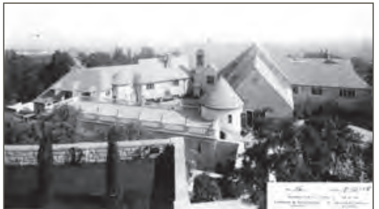
Construction Photo No. 11 Taken 9-12-28
