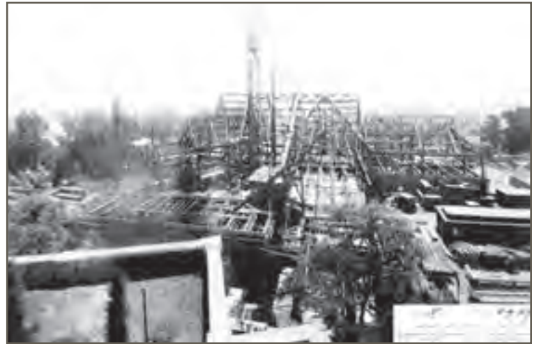
Construction Photo No. 5 Taken 8-9-27
