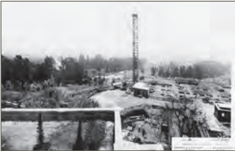
Construction Photo No. 2 Taken 5-9-27
