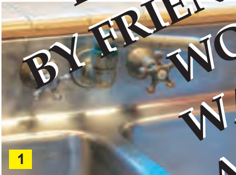
#1 The faucets in the flower room, kitchen and butler's pantry shall be re-plated. The cabinet hardware shall be replaced in the style of the original pulls, it is a fluted Drum shape knob 1920-40's style (there are numerous knobs missing and mixed designs presently).
