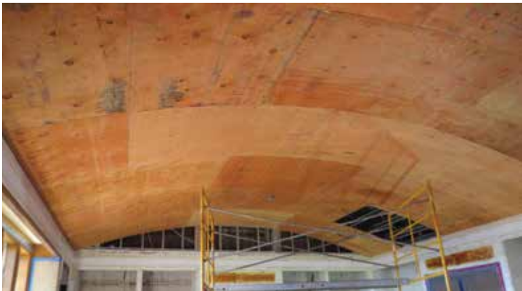
Barrell ceiling made with plywood
