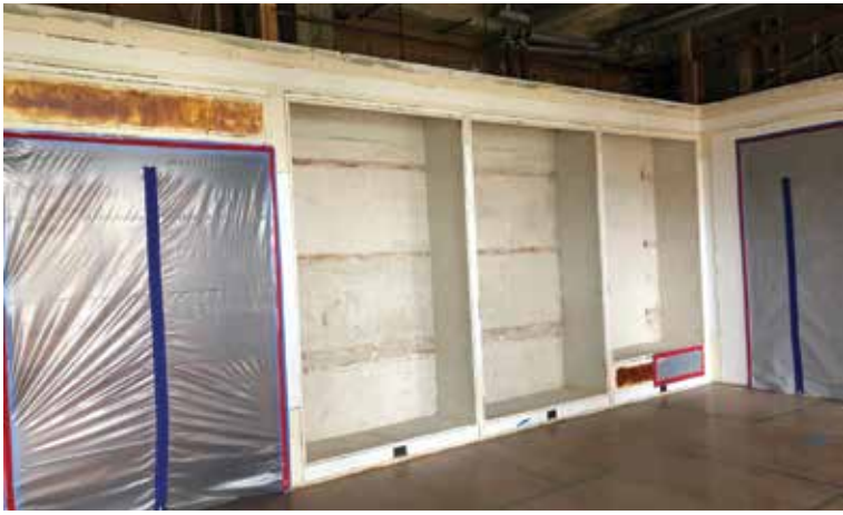
Bookshelves after demolition
