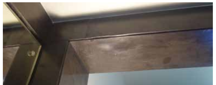
AFTER RESTORATION CHIPPED STONE REPAIRED
