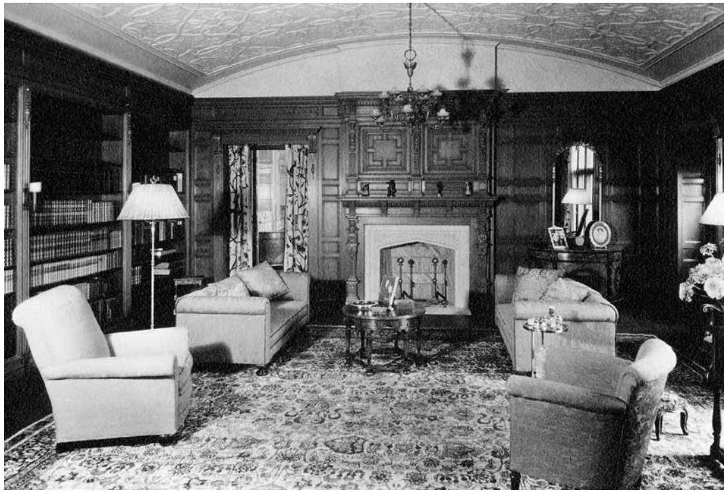
Doheny Greystone Mansion Library in 1928 and inspiration for current restoration
