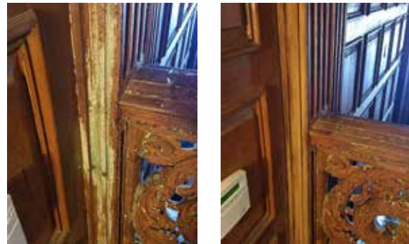
The photo on the left shows remnants of the historic paint layer applied by Mrs. Doheny Battson in the 1940s. The photo on the right shows the same area after the paint has been removed.
