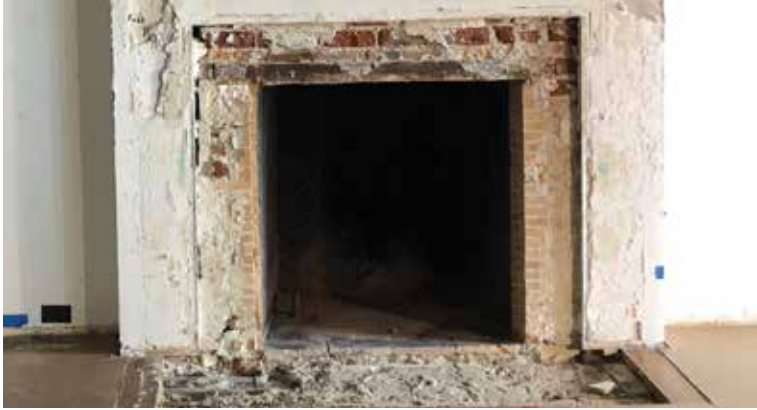
Fireplace after demolition
