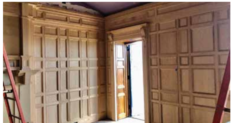
Wood panelling covering blank walls
