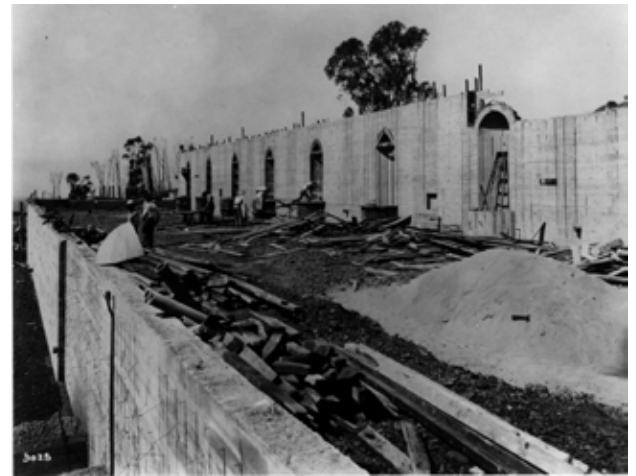
Cypress Lane under construction in 1927
